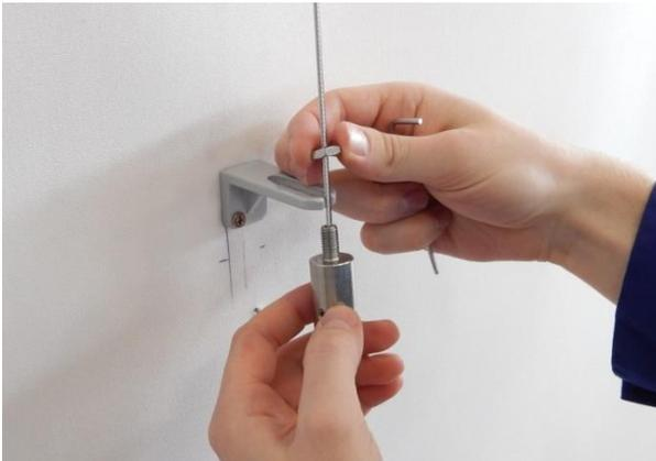
6. Install façade tightener to the bracket.
