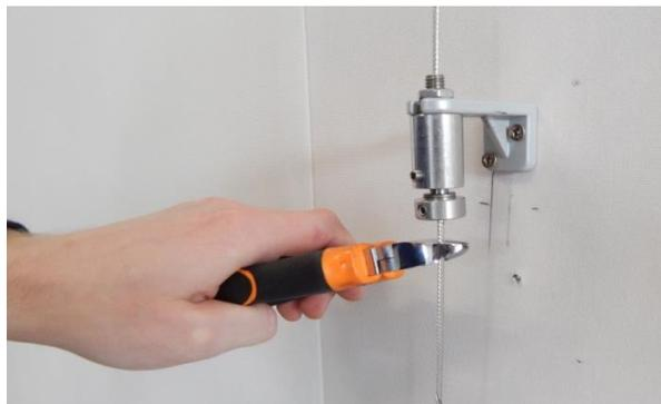
9. Cut out the excess of the cable.
