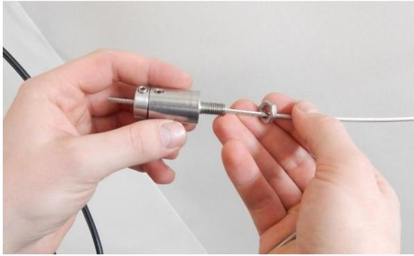
5. Put cable through façade tightener.
