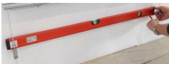
10. With a spirit level mark the installation place of the second cable guide bracket. Other actions perform analogically to the first bracket and guide.
