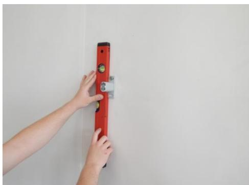
3. Check levels of the brackets, if needed correct it and secure the brackets.
