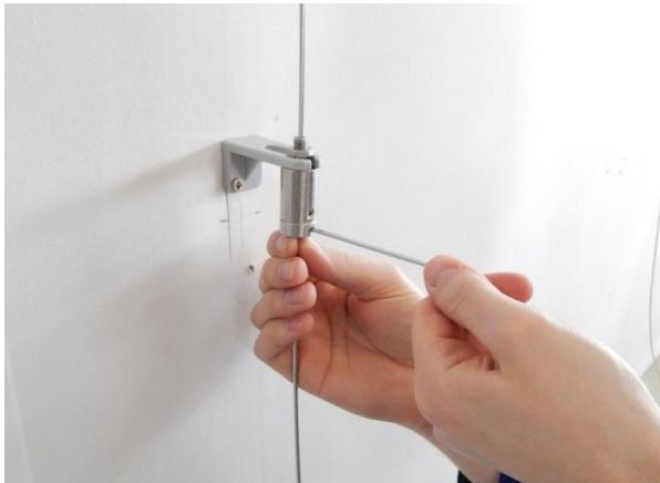
7. Secure the cable in tightener by tightening bottom screw until first resistance then use allen key and make 1,25-1,5 turn, remembering to leave some clearance required for correct tightener functioning. Exceeding the scope given will cause breaking the head, the screw slot or key head.
