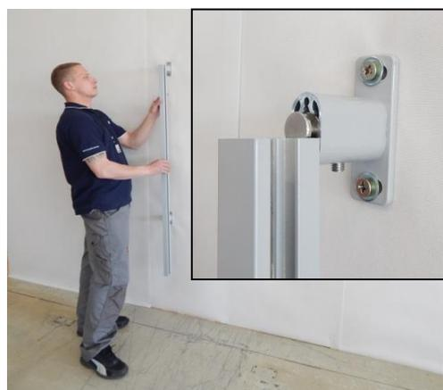
7. Slide the guide rails with rear profile onto the bolts.
